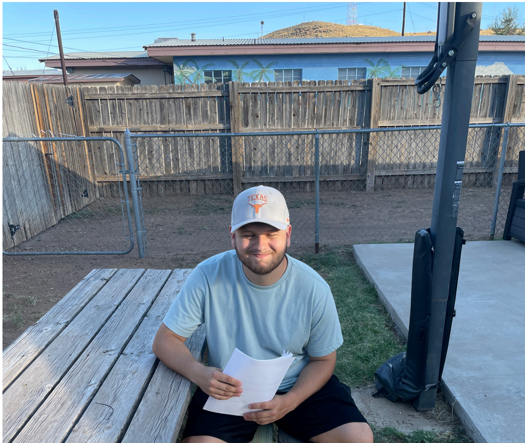
Chris is smiling because he just finished improving the bench near the basketball court. The rotten board is no more!
